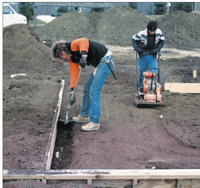
Figure 3. Slabs and footings for unheated buildings, such as the attached garage shown here, are placed directly on top of the foam insulation, with a foot of gravel under the foam. Stakes for the footing forms are driven through the foam (above). A trench is hand-dug inside the perimeter to form the slab's thickened edge (right).
